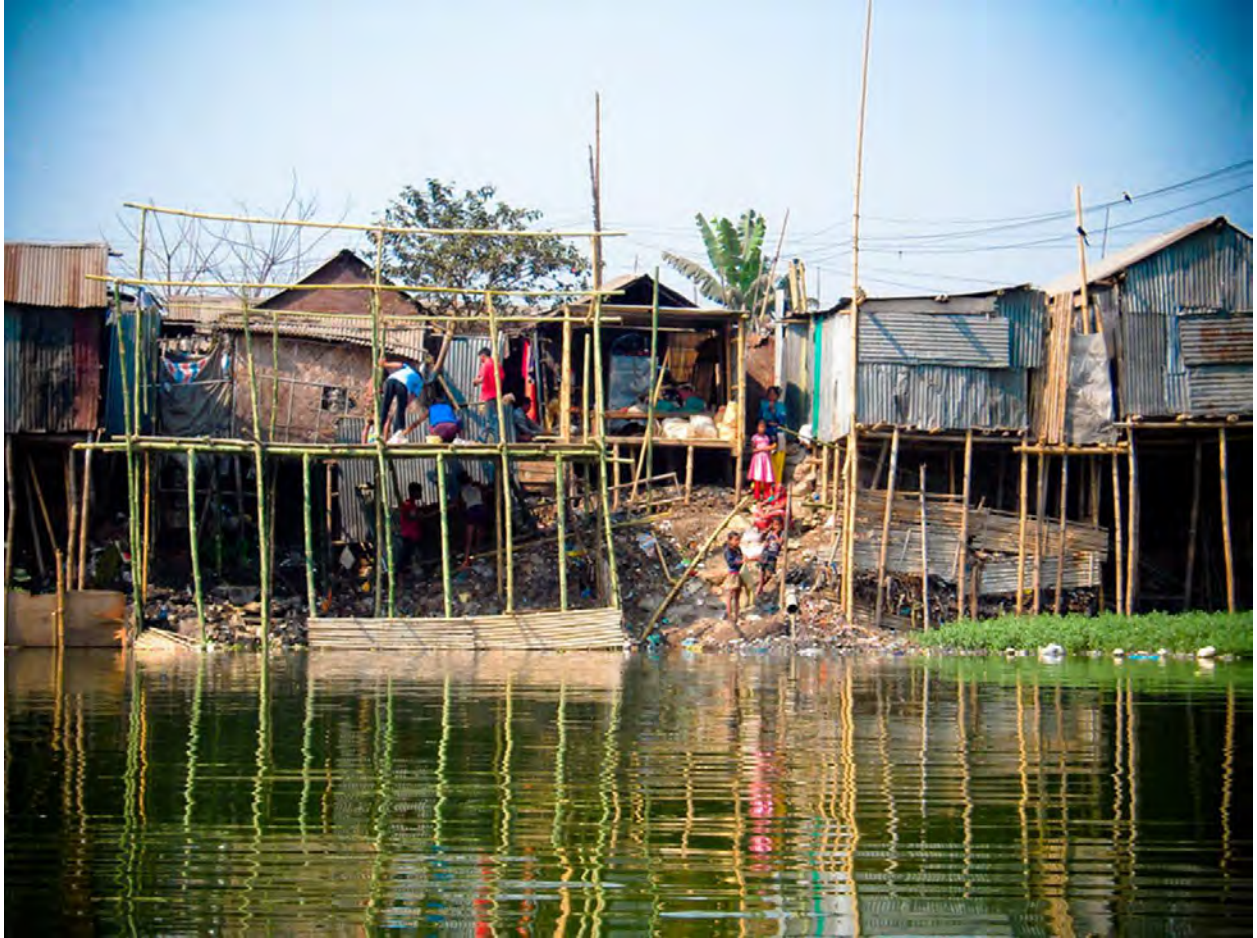
Bangladeshi people building houses on stilts so their homes are protected from flooding.
